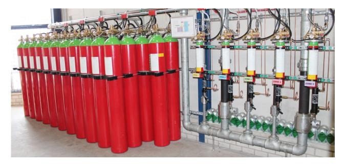
Equipment safe: Unlike many other agents that can become corrosive and permanently damage electronic components, Inergen does not form any corrosive by-products that can damage equipment in server rooms, data centres, medical facilities, laboratories or other sensitive electronic environments.
